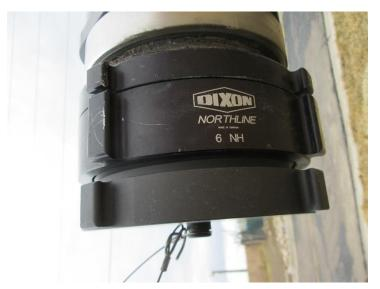
C. Secondary connection or "tank fill port" shall be a 2.5" NH Female swivel connection with cap and an additional cam-lock connection.
